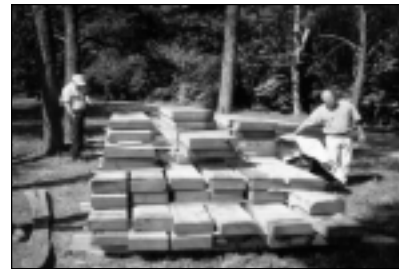
Good Wood. The new lumber for the repair work at Peirce Mill was milled recently at a lumber mill near Amherst, VA.
