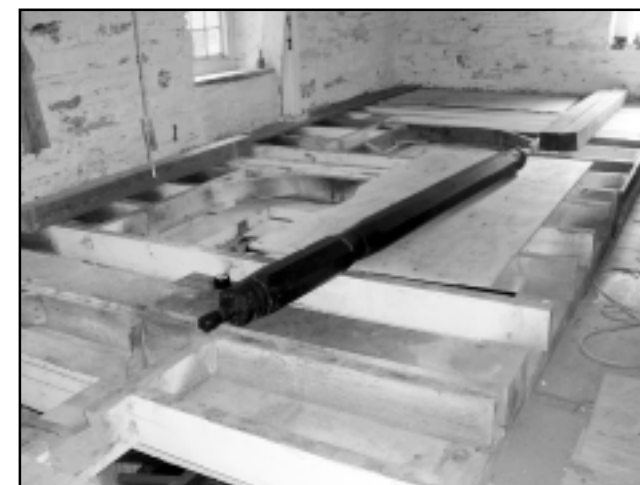
Millstones and millstone floor removed for repairs to hurst frame.
